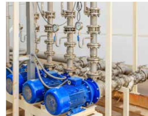
Sealing of flange connection
