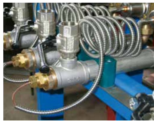
Bonding and sealing of pipe threads
