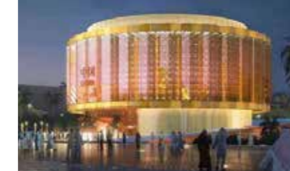
Project: Flexible LED curtain for EXPO 2020
